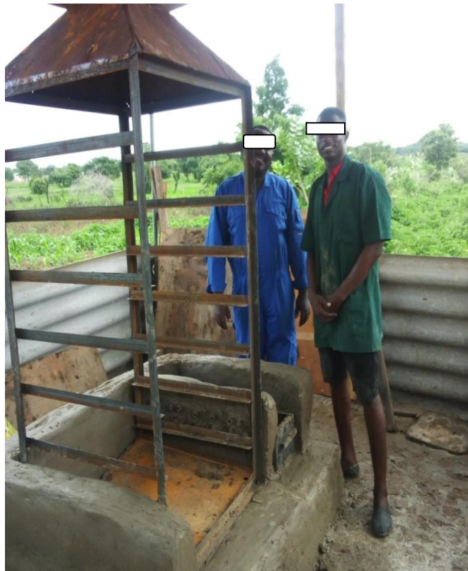
Plate 1. Kiln wall under construction
