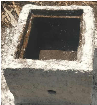
11.Repairs and Cleaning
