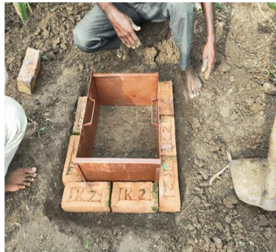
5. Iron plank and Frame Placement
