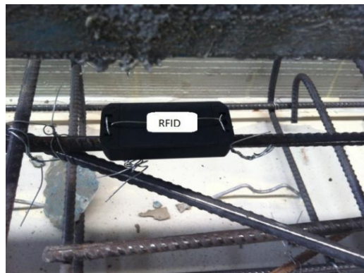
Fig. 10. RFID chip is embedded in the component
