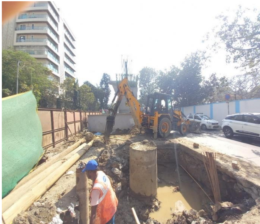
Fig. 2. Backhoe Loader with Drill attachment
